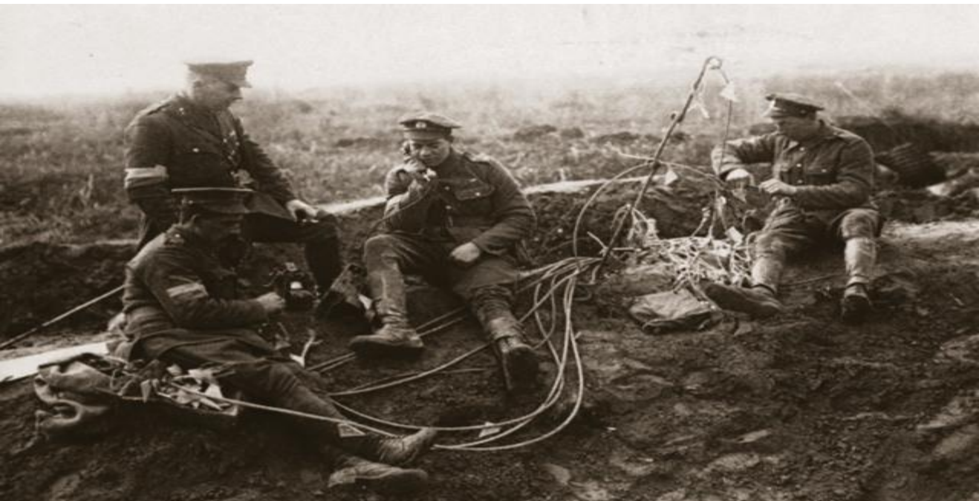
Royal Engineers instalando linhas telefónicas (Flandres, 1917)
